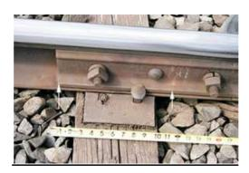
Creep in rails denotes longitudinal movement of rails in the track.
