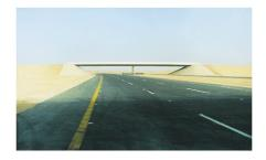
Already used for lengths up to 60m, the integral bridge is becoming increasingly popular as engineers and designers find other ways of dealing with thermal movement.
