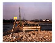
Simply supported concrete beams and slab bridges are now giving way to integral bridges which offer the advantages of less cost and lower maintenance due to the elimination of expansion joints and bearings.
